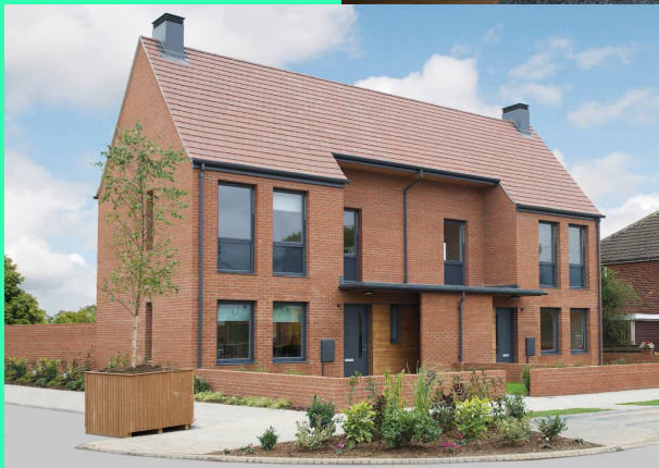
This development used fully reversible windows with coloured opaque glass on the first floor.
