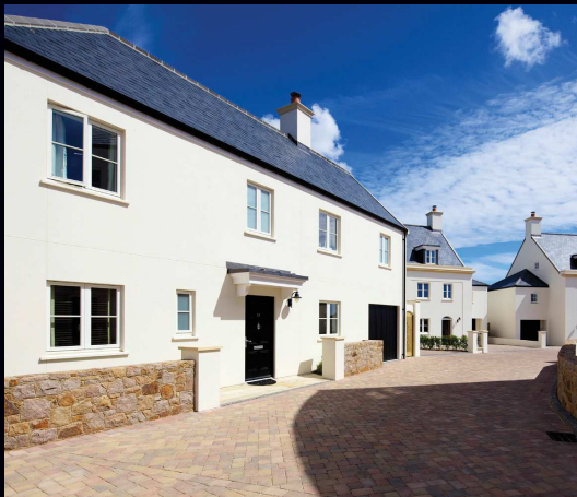
This residential development used sideguided windows with horizontal glazing bar
